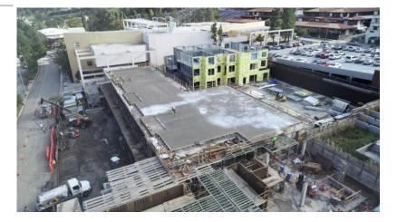
MERRILL GARDENS AT WEST COVINA: Crews in West Covina have completed the ground improvement work with the installation of more than 500 geo piers and are now making progress on the building foundations. The construction team's focus for the next month will be completing the concrete footings and working on underground mechanical, electrical and plumbing work. This project is scheduled to be complete in the 2nd quarter of 2020.
