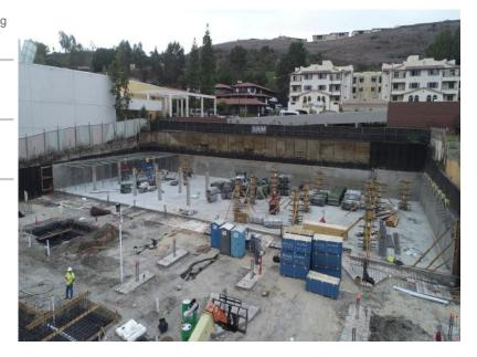
**WESTMONT OF MILPITAS** - Westmont of Milpitas is out of the ground and moving up. During the month of September, the remaining slab on grade pours were completed and work on the PT decks has moved along rapidly. The first half of the Level 2 transfer slab is on schedule to be complete and ready for wall panels by the end of November and we are looking forward to having a good jump on framing by years end. Keep up the good work, Team Milpitas!
